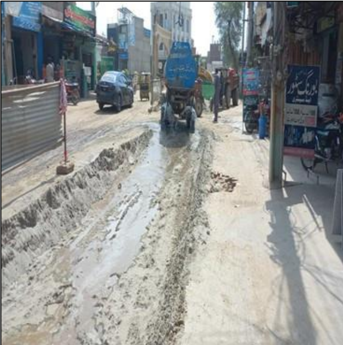
Picture 14: Sprinkling and Spreading of Sand at L-2.5 42" Dia.
