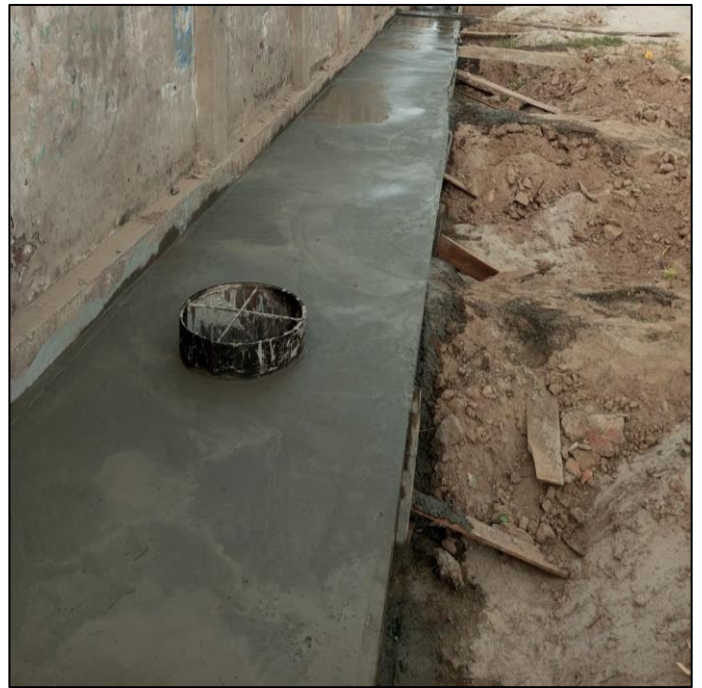
Picture 64: Drain RCC Slab at Iqbal Road
