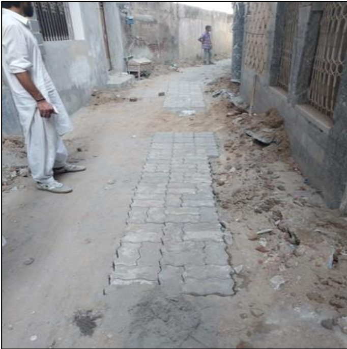
Picture 48: Restoration of tuff pavers
