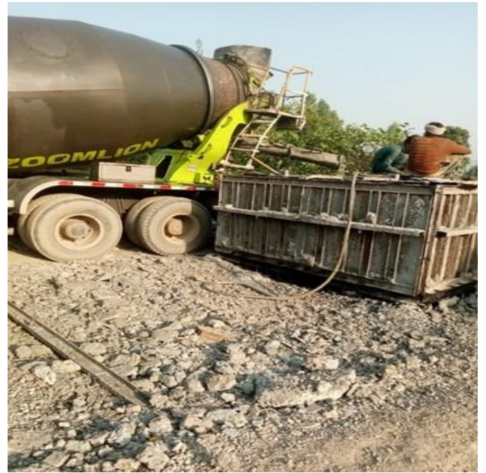
Picture 35: Conduit Pouring in Progress at ZKB Camp
