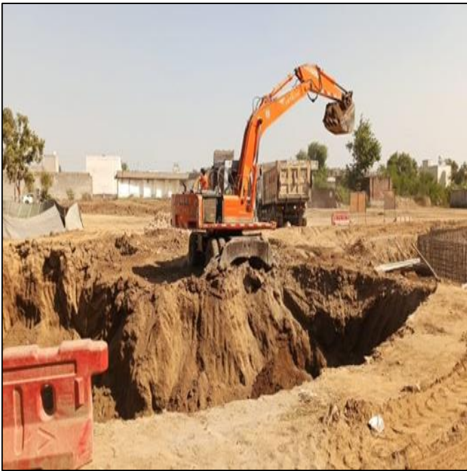
Picture 46: Excavation of Dry Well
