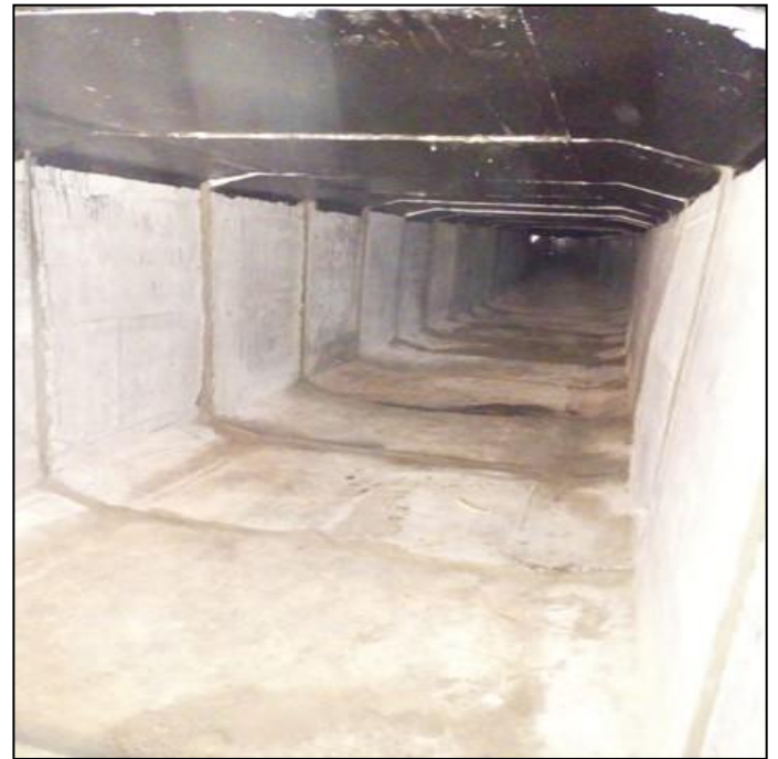
Picture 39: Internal Conduits after Cleaning at Marala Road
