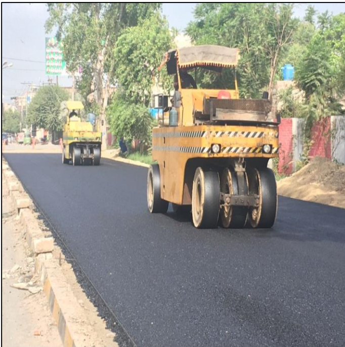
Picture 59: Compaction of Asphalt Base Course
