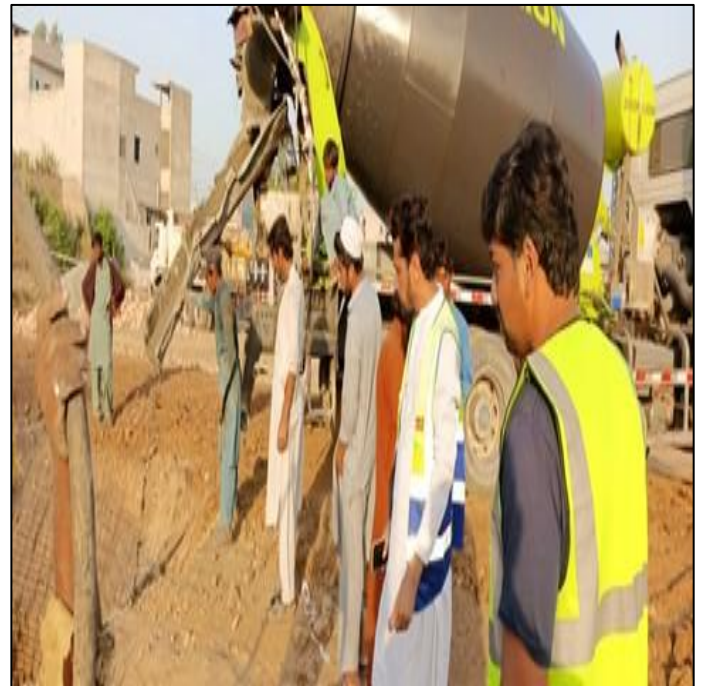
Picture 43: Concrete of Wet Well
