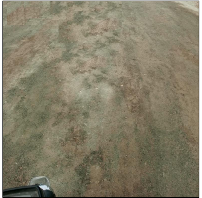
Picture 62: Aggregate Base Course Leveling Layer at High Street Road
