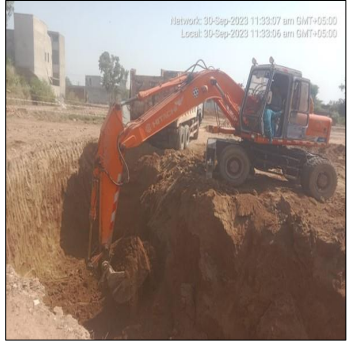
Picture 45: Excavation of Dry Well
