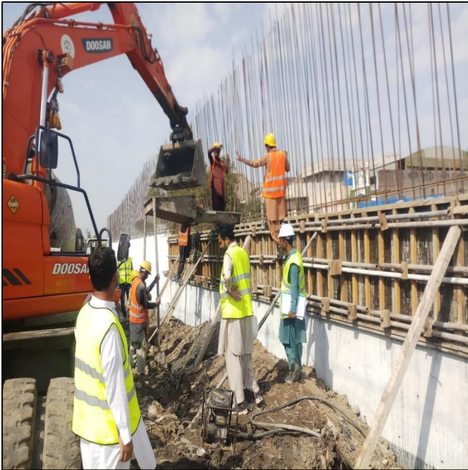
Picture 69: Pouring of Retaining Wall Concrete is in Progress
