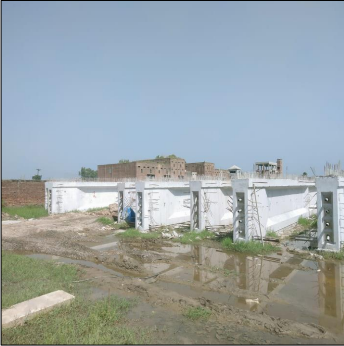
Picture 77: Views of Casted Girders
