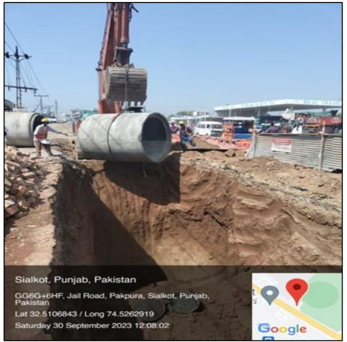
Picture 29: RCC 72" Dia. Sewer Laying in Progress @ Lari Adda Road
