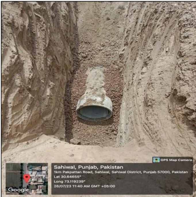
Picture 22: Laying of 36-inch dia pipe in progress at Pakpattan Road
