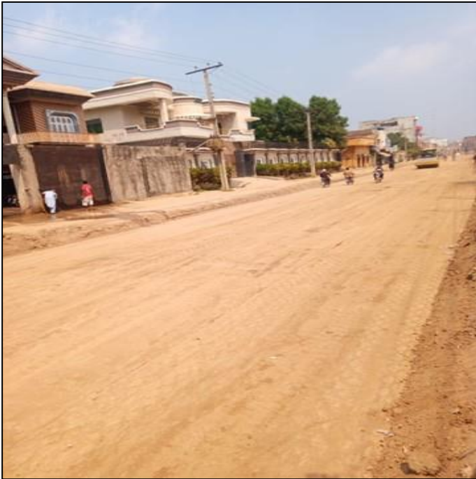
Picture 40: Subgrade 1st Working in progress at Marala Road
