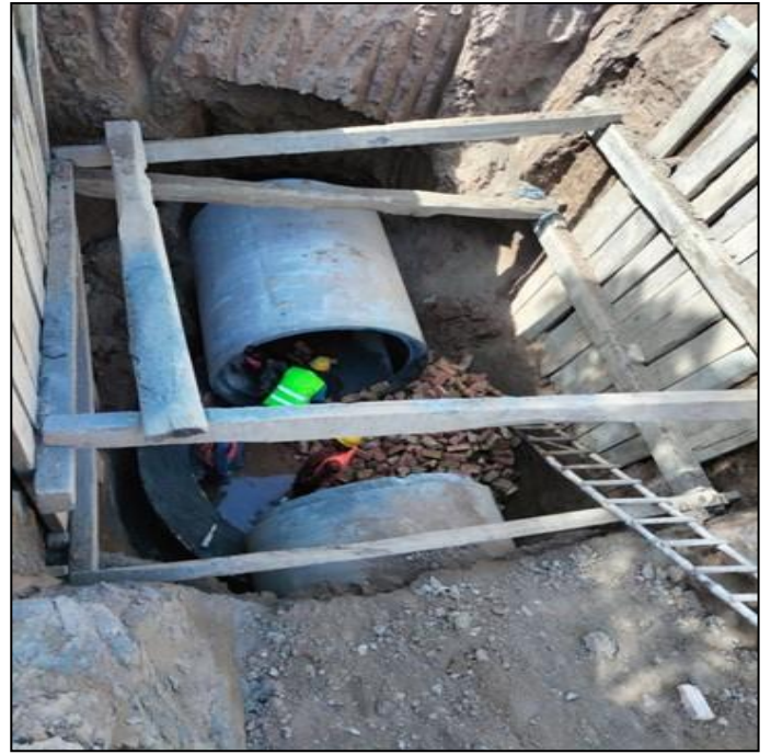
Picture 33: MH 92 Brickwork in Progress @ Lari Adda Road
