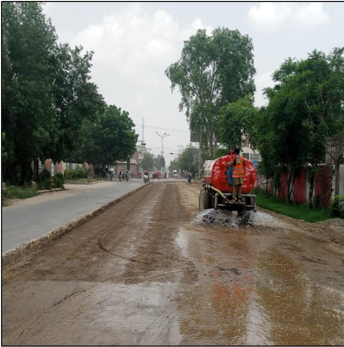
Picture 61: Compaction for Aggregate base Course Leveling Layer
