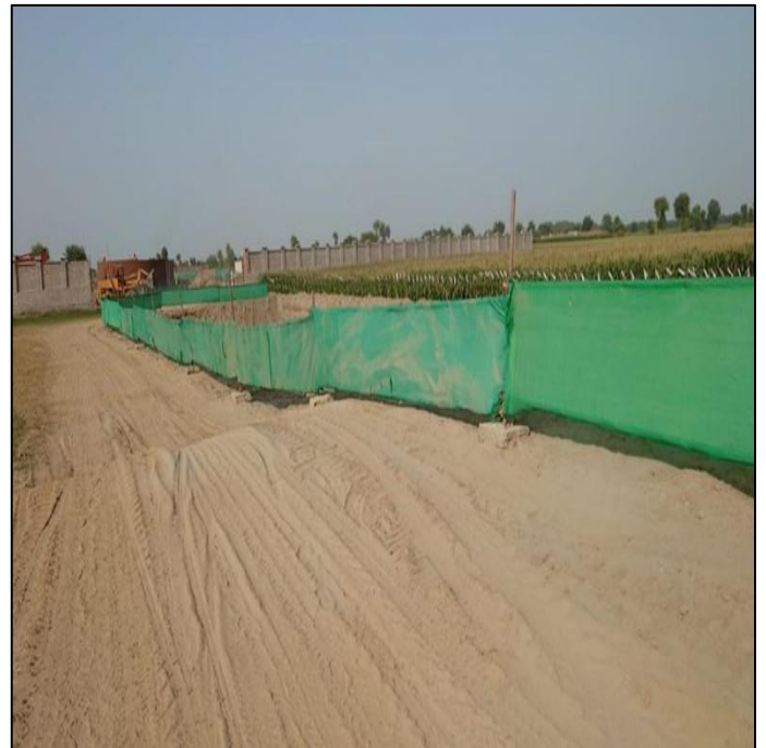
Picture 17: Spreading of Subbase at L 2 48" Dia in progress
