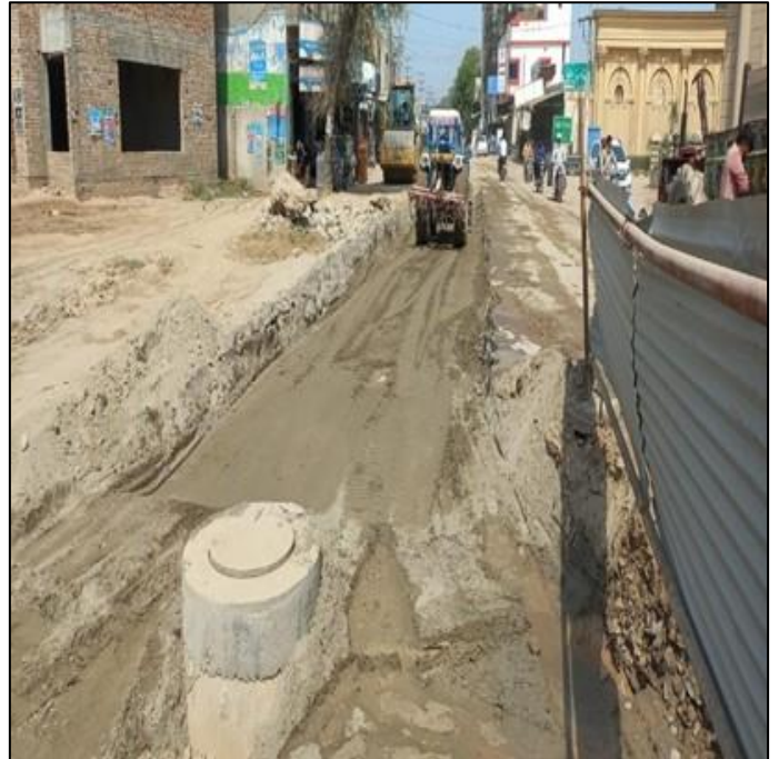
Picture 15: Sprinkling and Spreading of Sand at L-2.5 42" Dia
