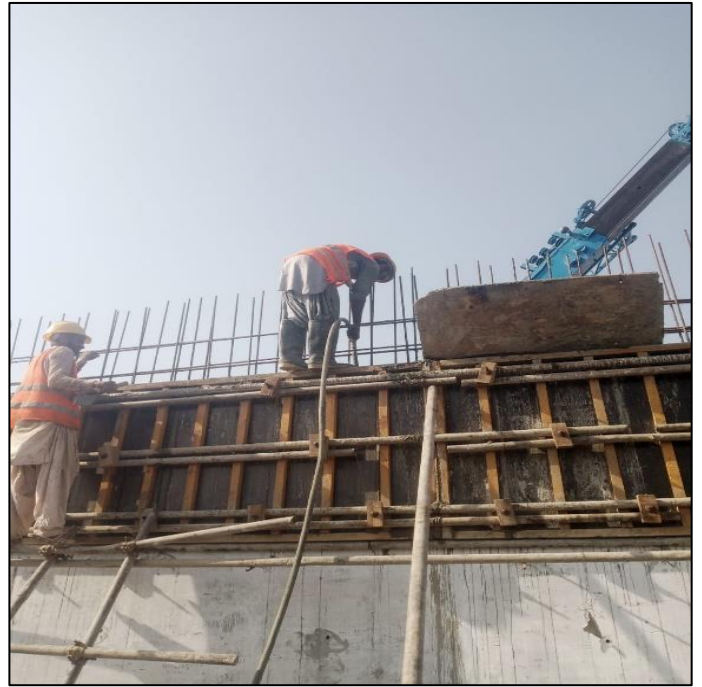
Picture 74: Pouring of Retaining Wall Concrete is in Progress
