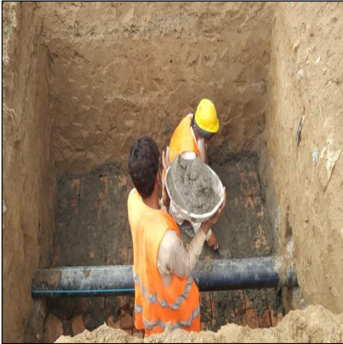
Picture 8: : Construction of sluice valve UC-04
