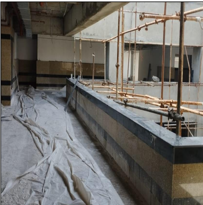
Picture 53: Fixing of Granite Tiles at Walls and Parapet
