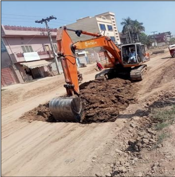
Picture 34: Removal of Slush Point at Marala Road
