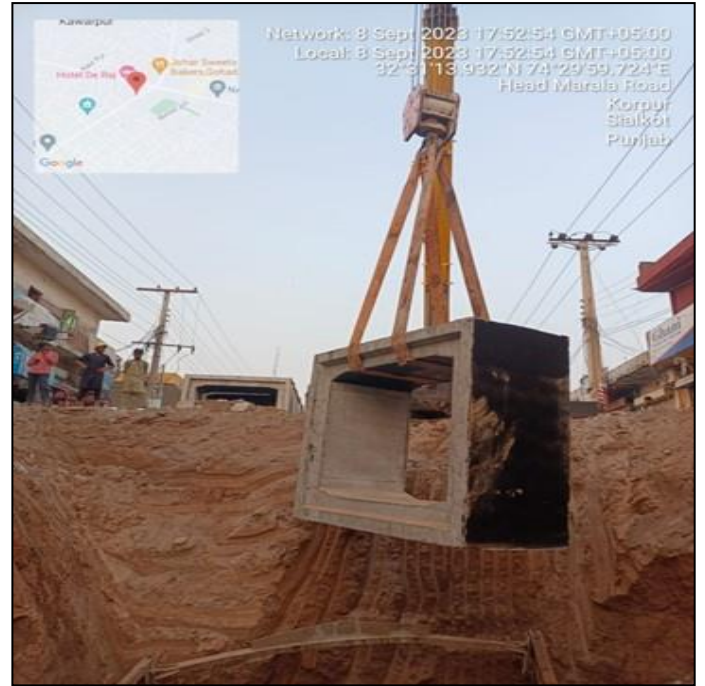
Picture 37: Single Cell Conduit Laying @ Marala Road
