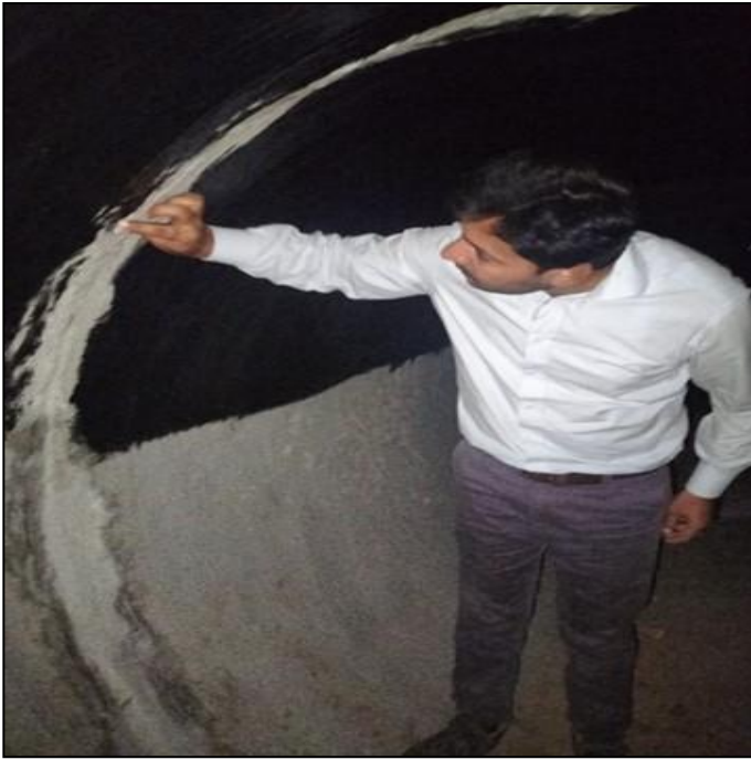
Picture 32: 72" Dia. Pipe Internal Joint Verification in Progress @ Lari Adda Road
