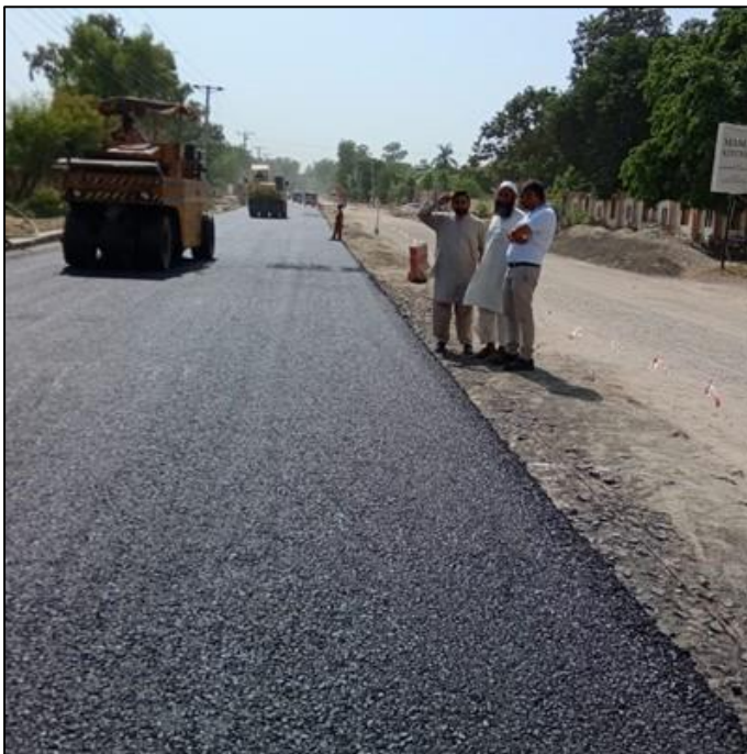
Picture 26: TST in progress
