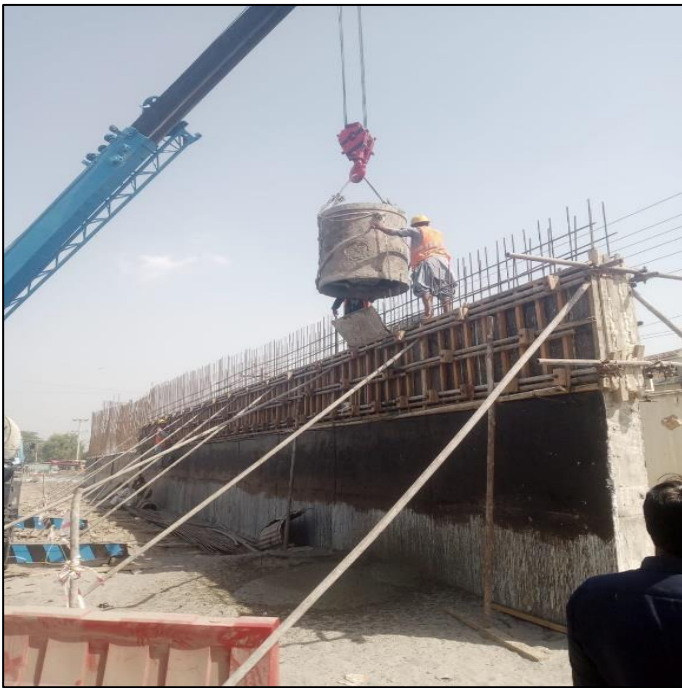
Picture 75: Pouring of Retaining Wall Concrete is in Progress
