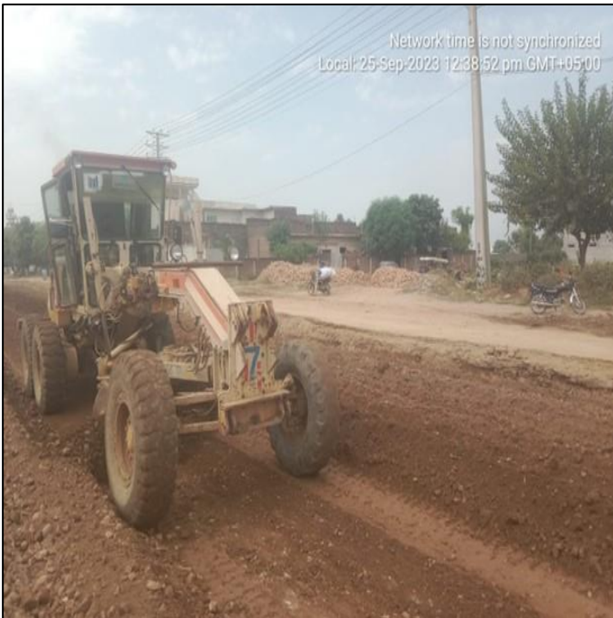
Picture 42: Road Restoration of Force-main Site
