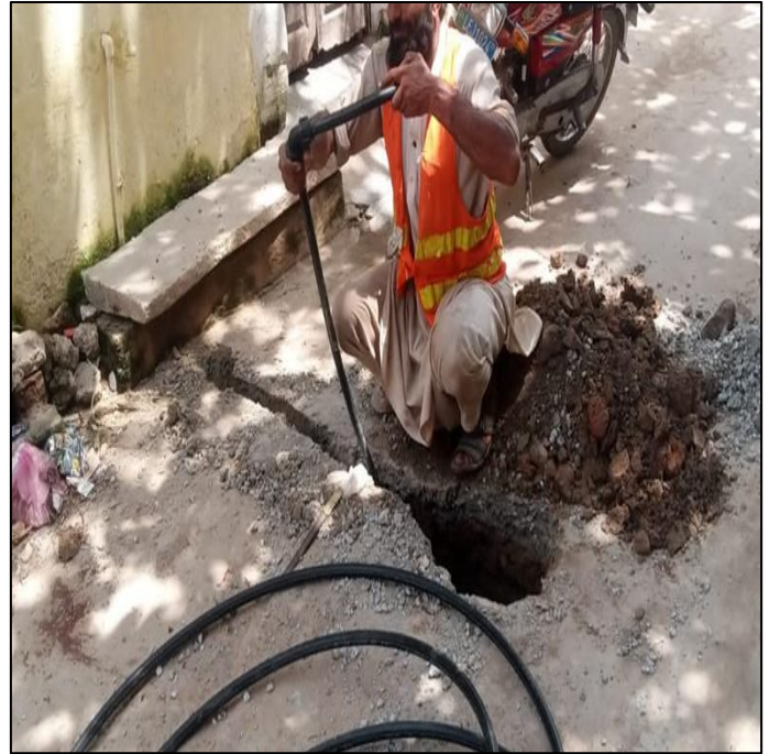
Picture 9: Fixing of House Connection UC-6
