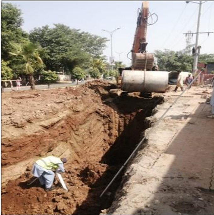
Picture 30: 54" Dia. Pipe Laying in Progress @ Khawaja Safdar Road
