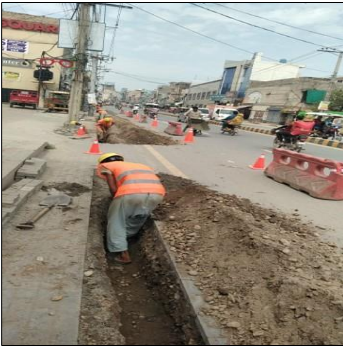
Picture 50: Pipe laying works along Khadim Ali Road
