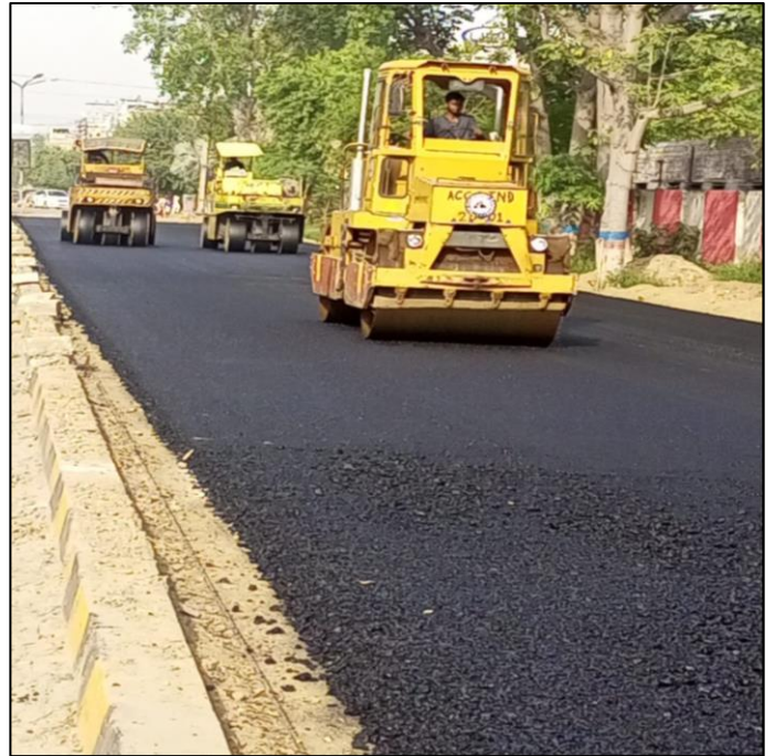
Picture 58: Compaction of Asphalt Base Course
