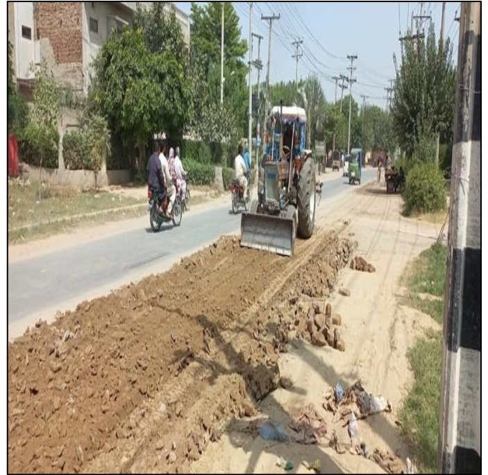
Picture 17: Spreading of Subbase at L 2 48" Dia in progress
