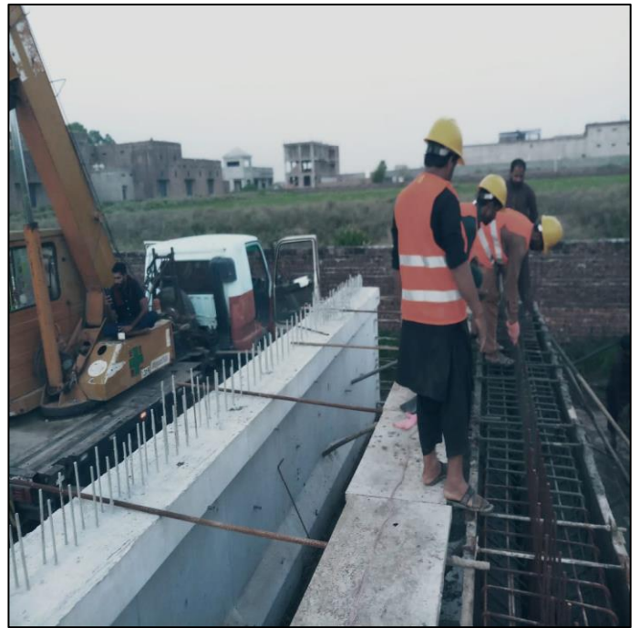
Picture 80: Pouring of Girder Concrete in Progress
