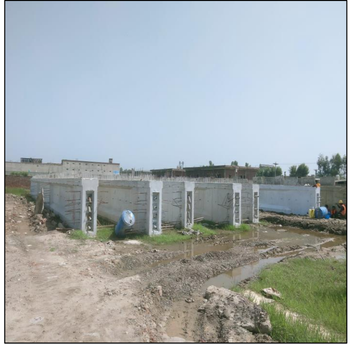
Picture 78: Views of Casted Girders
