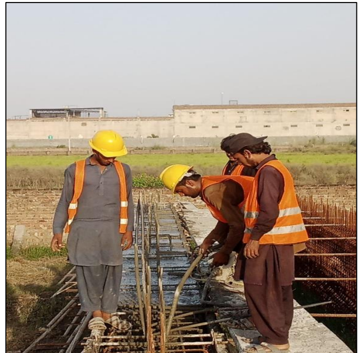
Picture 72: Profile Checking and Pouring of Girder Concrete in Progress
