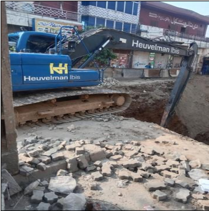
Picture 36: Excavation in Progress at Marala Road
