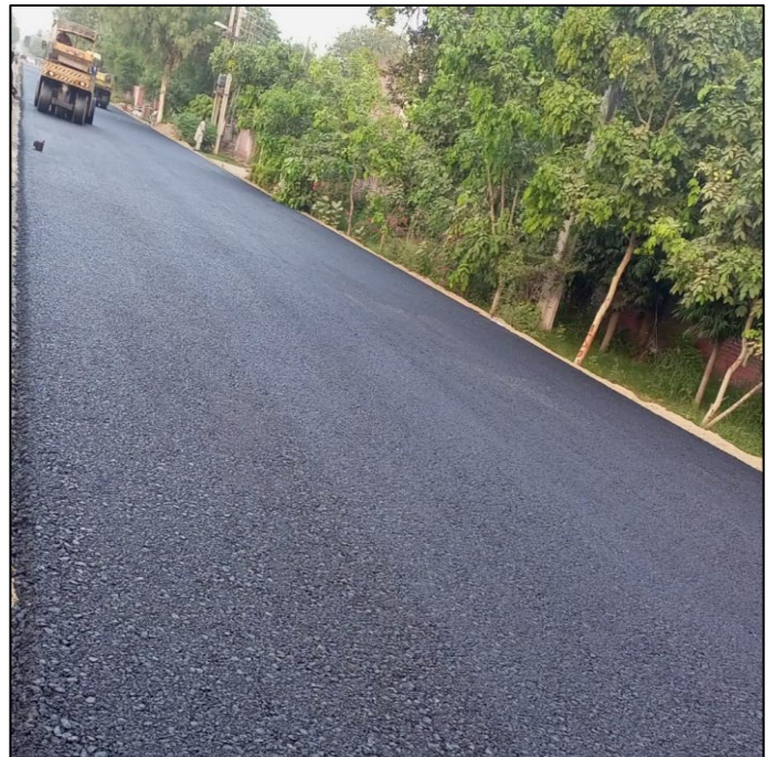
Picture 60: Asphalt Work in-progress at Iqbal Road L/S
