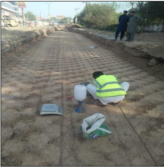
Picture 28: FDT in Progress @ Lari Adda Road
