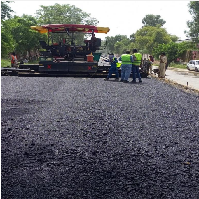
Picture 57: Paving of Asphalt Base Course at Iqbal Road
