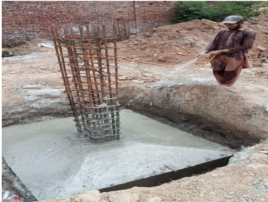
Picture 56: Concrete and Curing of RCC footing is in progress
