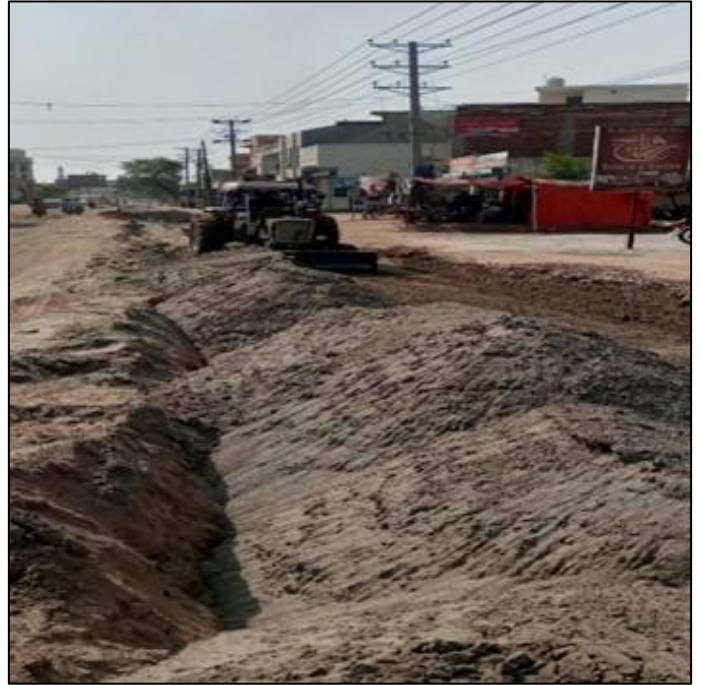
Picture 13: Filling of Sand at L-1.9.4.1 21" Dia in Progress
