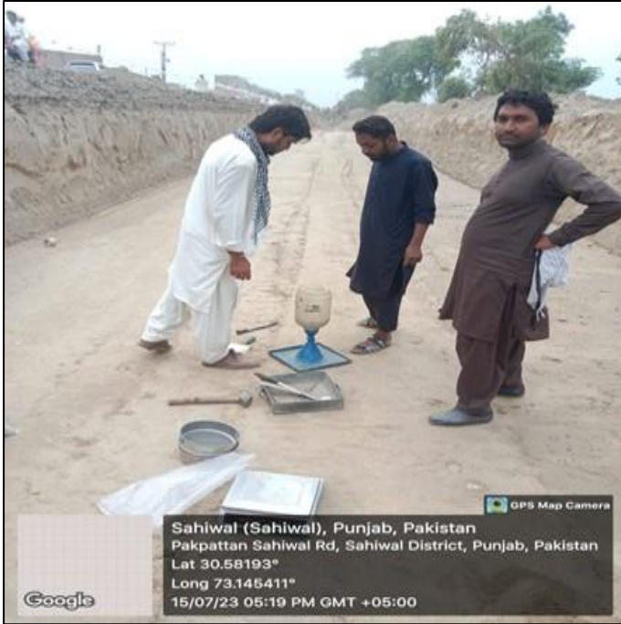
Picture 24: Field Density Test of Backfilled material
