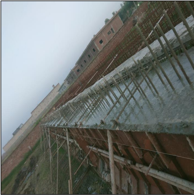
Picture 73: Pouring of Girder No 10 Concrete completed
