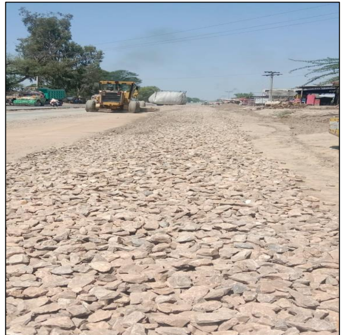
Picture 23: Restoration of Pakpattan Road in progress
