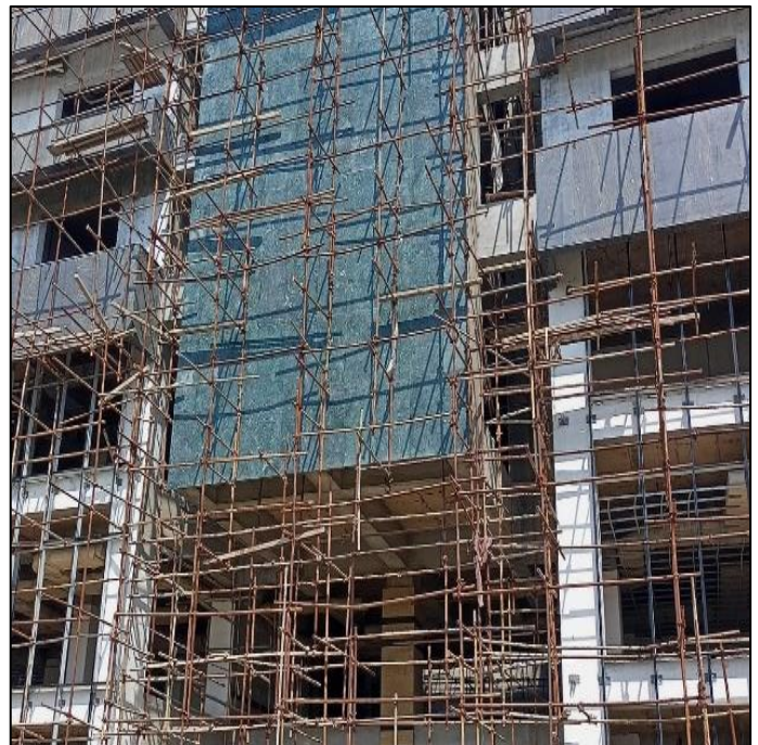
Picture 54: Fixing of Granite Tiles at Front Elevation
