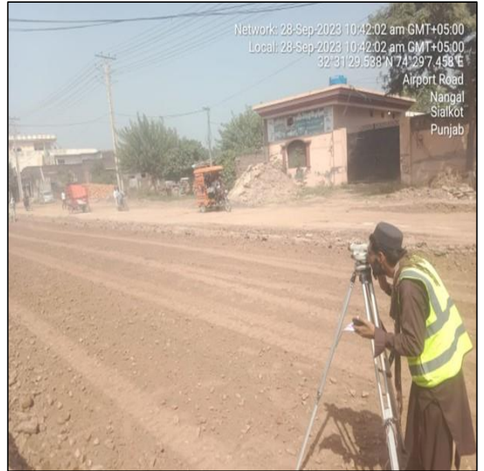
Picture 41: Road Restoration of Force-main Site
