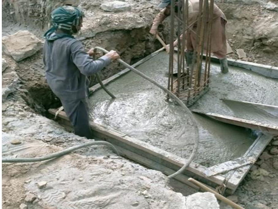
Picture 55: Concrete and Curing of RCC footing is in progress
