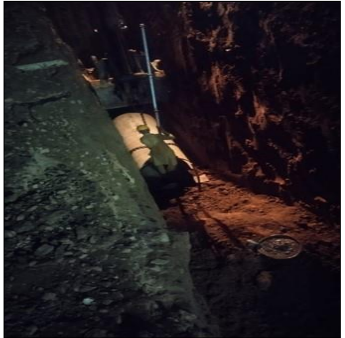
Picture 31: 33" Dia. Sewer Laying @ Paris Road
