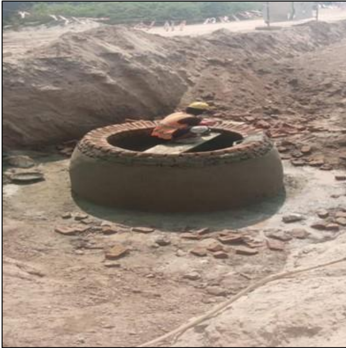
Picture 16: Construction of Manhole is in Progress
