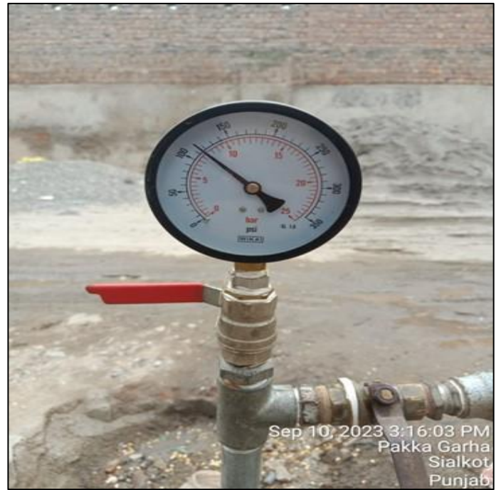
Picture 47: Pressure testing in progress
