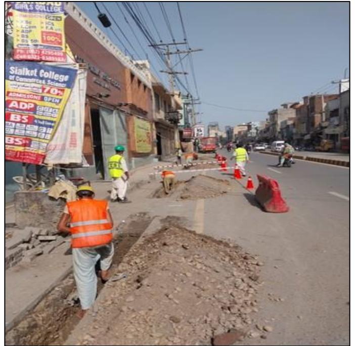
Picture 49: Pipe laying works along Khadim Ali Road
