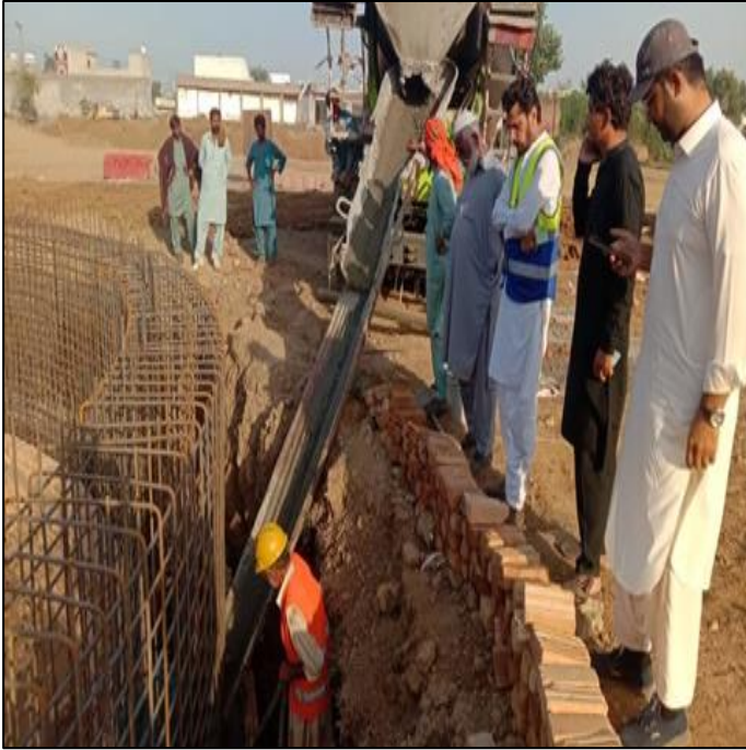
Picture 44: Concrete of Wet Well
