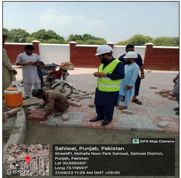
Picture 11: Concrete Tuff paver in progress at OHR T6
