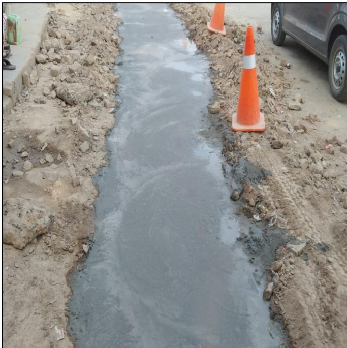
Picture 10: Restoration Work UC-10
