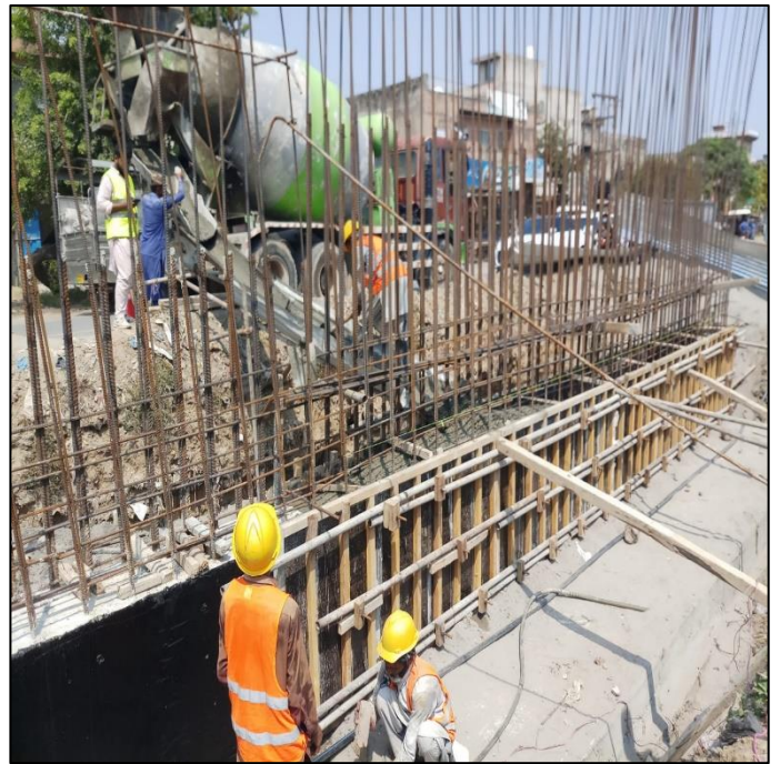
Picture 76: Pouring of Retaining Wall Concrete is in Progress
