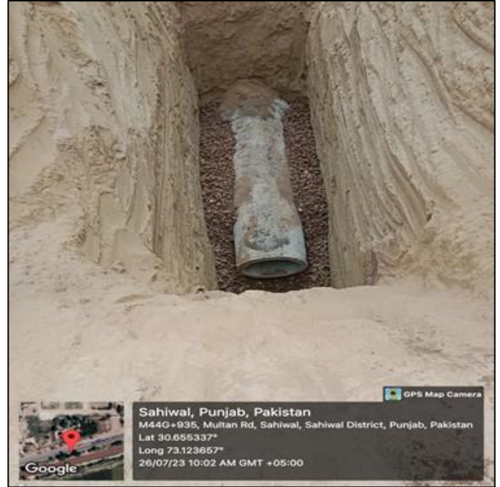
Picture 21: Laying of 21-inch pipe dia at Lahore Multan Road
