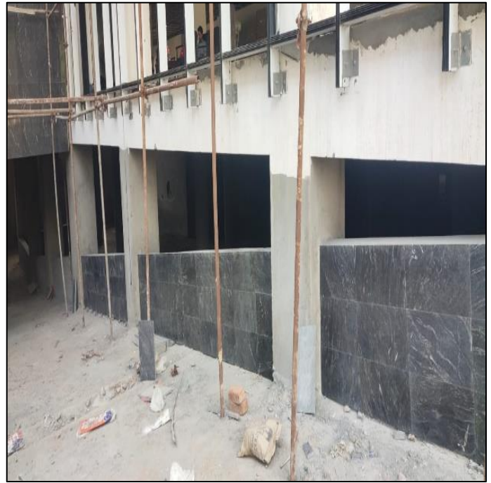
Picture 52: Fixing of Granite Tiles at Ramp Wall
