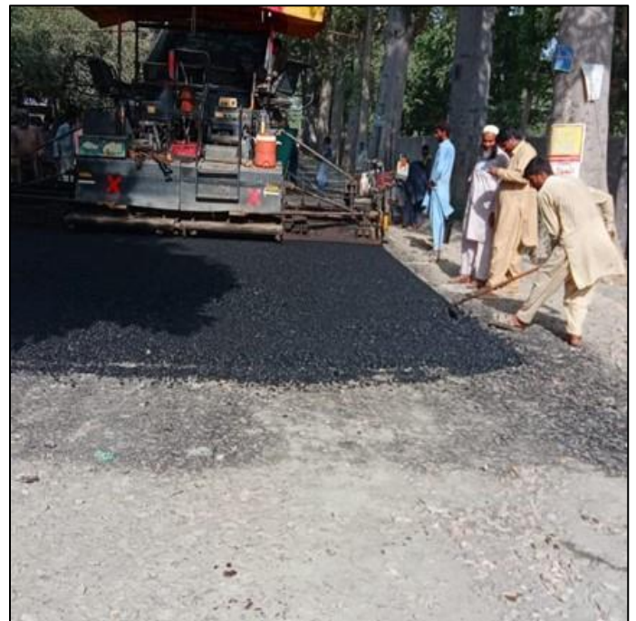
Picture 27: TST in progress
