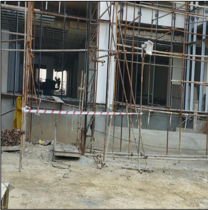
Picture 51: Shuttering view
